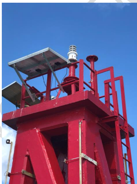
Figure 4: Prototype three-tiered Dual Intensity Lantern Installed on Cyrene Beacon for third onsite trial (Phase 3). (Fl.R.2,5s8m10M)
