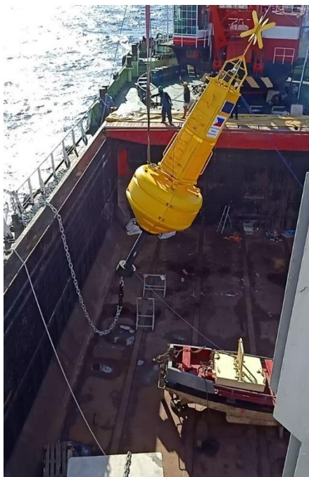
Figure 7: Lifting of a buoy from the Installation Vessel cargo hold.
