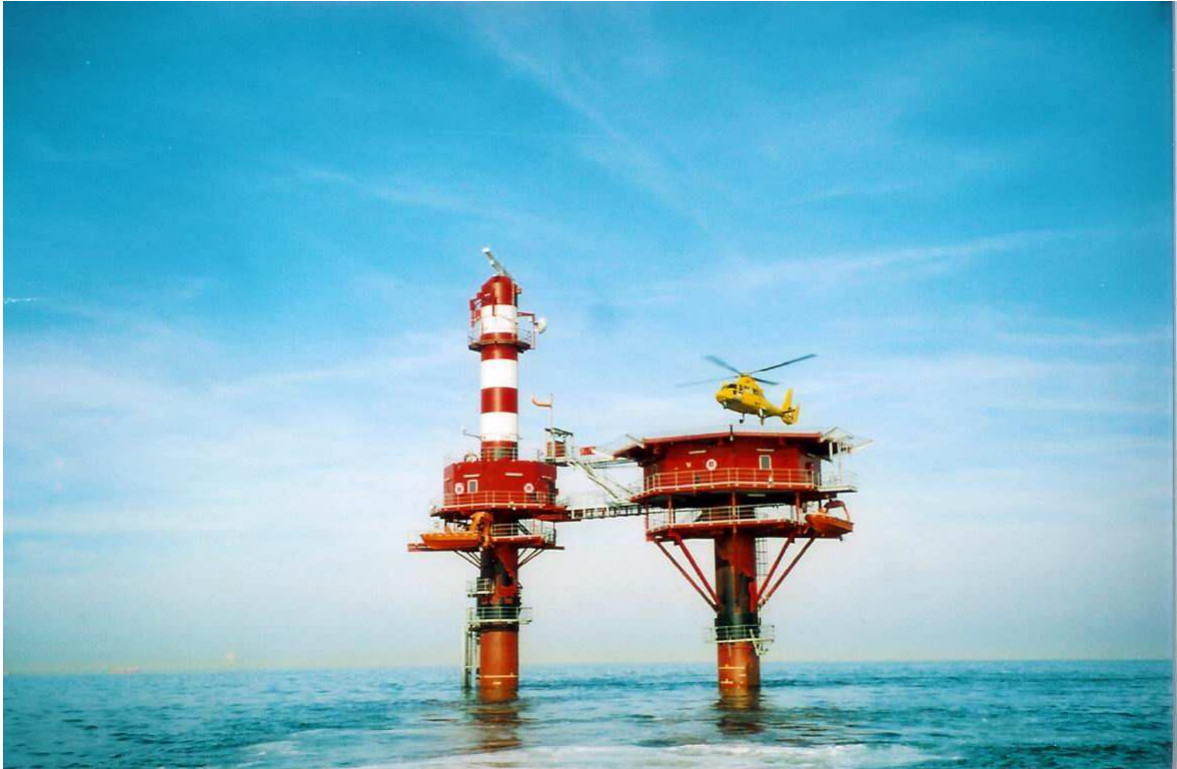
Radar is a key requirement for most VTS. Siting the antenna in the right location and obtaining adequate height requires much consideration. Some solutions: above, an automatic facility at Oostdyckbank, ten miles off the Belgian coast (Flemish Waterways); below left, at Saeftinghe, and below right, the old tower at La Maddalena, Italy. (Italian Coastguard)
