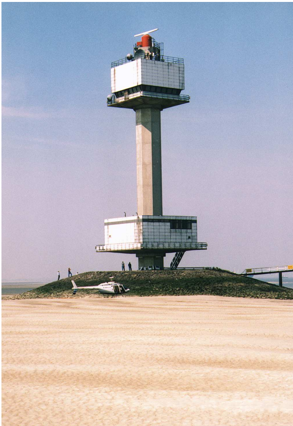
Radar is a key requirement for most VTS. Siting the antenna in the right location and obtaining adequate height requires much consideration. Some solutions: above, an automatic facility at Oostdyckbank, ten miles off the Belgian coast (Flemish Waterways); below left, at Saeftinghe, and below right, the old tower at La Maddalena, Italy. (Italian Coastguard)
