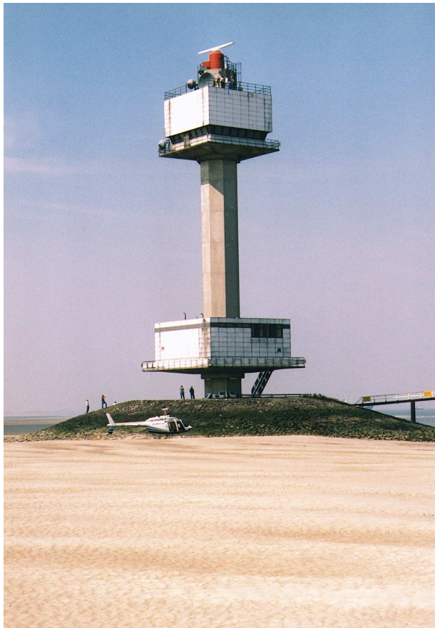
Radar is a key requirement for most VTS. Siting the antenna in the right location and obtaining adequate height requires much consideration. Some solutions: above, an automatic facility at Oostdyckbank, ten miles off the Belgian coast (Flemish Waterways); below left, at Saeftinghe, and below right, the old tower at La Maddalena, Italy. (Italian Coastguard)
