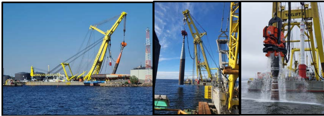
Figure 2. The transportation (left) and installation (middle and right) of the base piles was carried out by a special vessel TAKLIFT 4 (Home Port: Rotterdam, Flag: Singapore).
