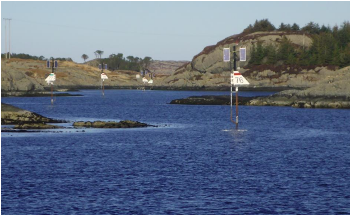
Figure 9 Day-time view - indirect lighting used on beacons in Norwegian waters
