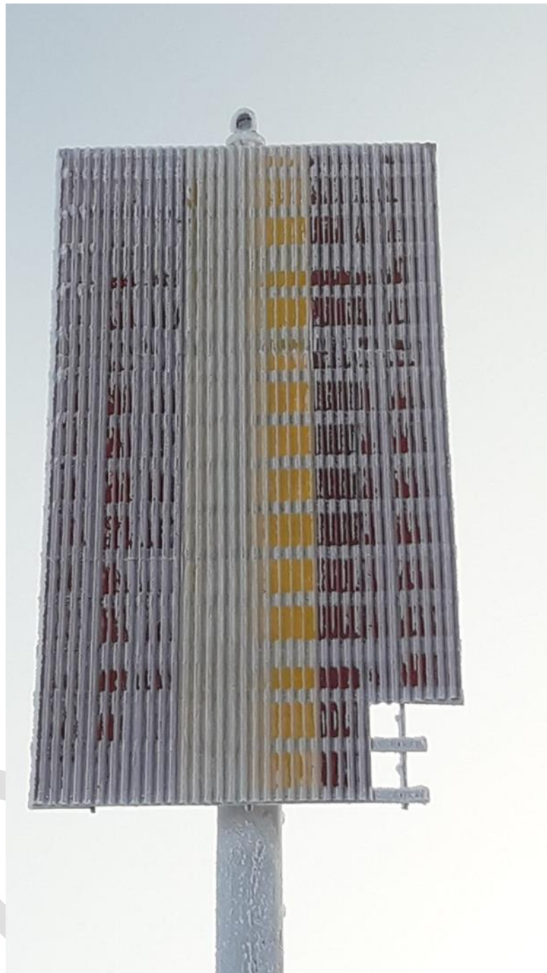
Figure 7 Leading light (and dayboard) covered in ice
