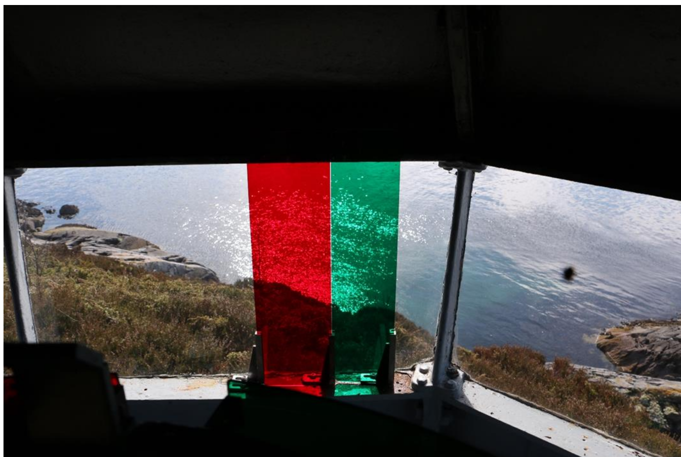
Figure 3 Sector filters fitted inside a lighthouse lantern
