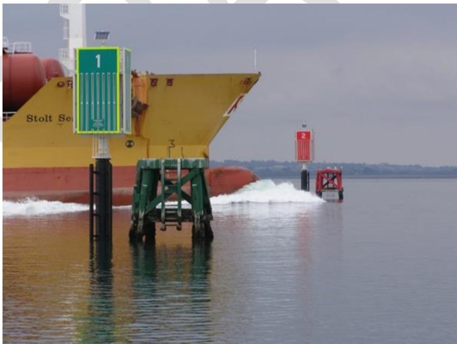
Figure 10 Advantage of solid shape as opposed to “see through”
