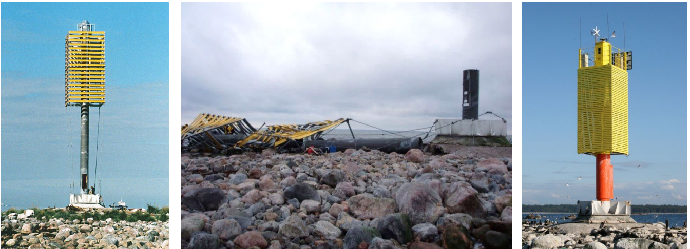
Figure 12 Aegna Island northern light – (left to right) original, destroyed and replacement
