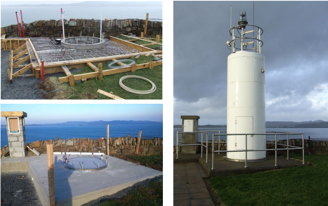
Figure 11 Example of GRP light tower and foundation base, during and after construction
