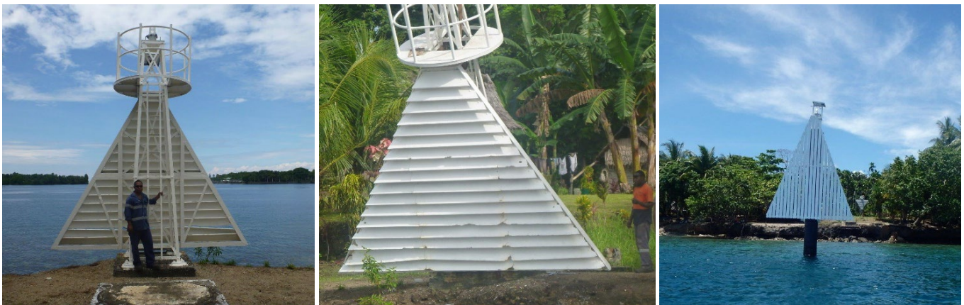
Figure 13 Front Lead dayboard and light – (left to right) rear and front view of land sited light and monopile replacement
