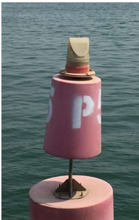
Figure 30 High Ultraviolet effect on red buoy
