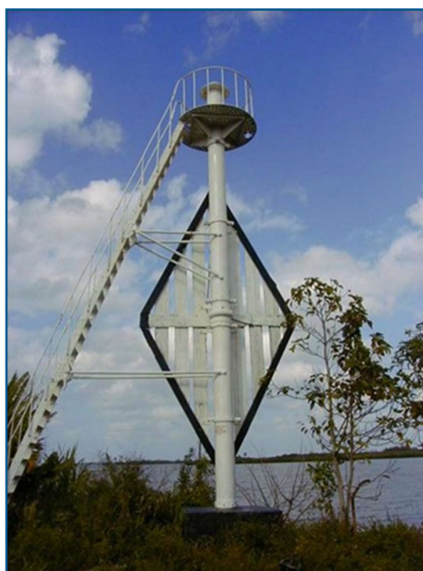
Figure 2 Front leading light with daymark lattice design
