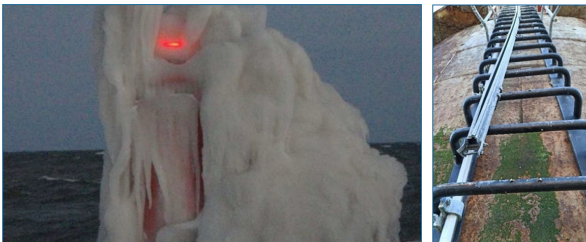
Figure 13 Port entrance mark covered by ice – safety rail bent by ice on Tallinnamadal lighthouse
