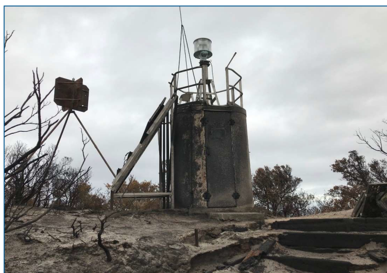
Figure 21 Example of AtoN destroyed by fire
