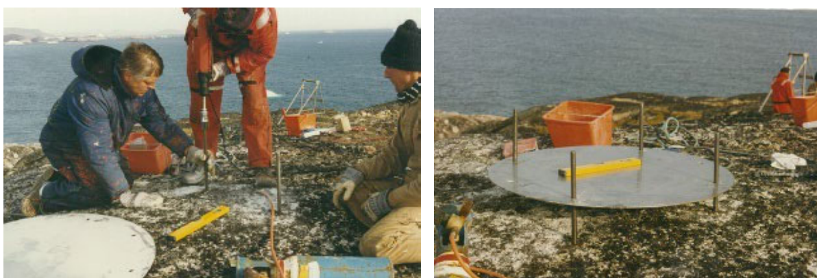
Figure 14 Examples of a simple foundation which is preferred in Polar Regions to ensure a swift installation and to reduce the use of heavy equipment and large quantities of material 1
