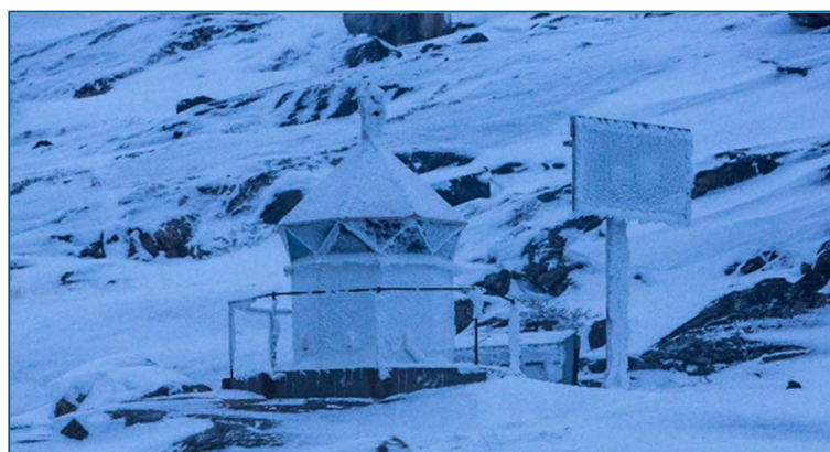
Figure 12 Example of ice on AtoN structure
