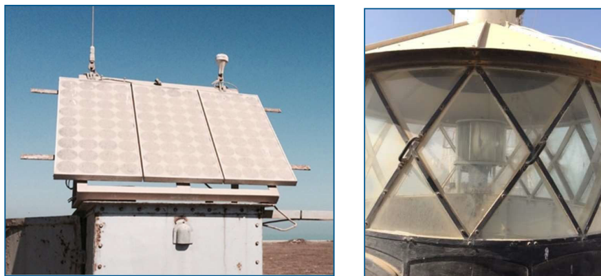
Figure 19 Presence of dust on AtoN device
