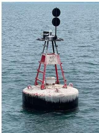
Figure 17 Example of guano on floating AtoN (an Isolated Danger Mark)
